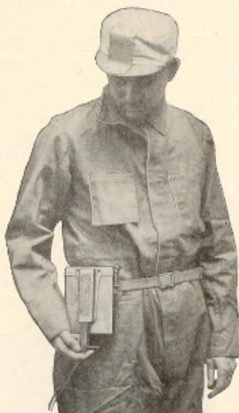
Edison Shot-Firing Battery. Showing how special cover for shot-firing is attached to regular Edison Mine Lamp.
