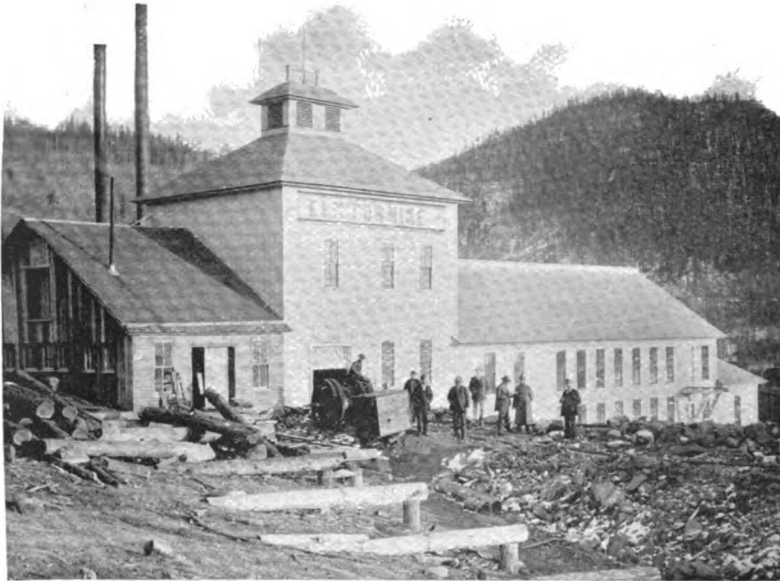
THE ELKTON SHAFT HOUSE
