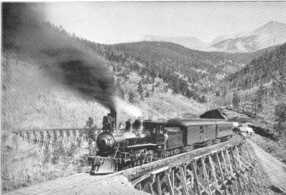
CIRCULAR TRESTLE. On Midland Terminal Railroad.
