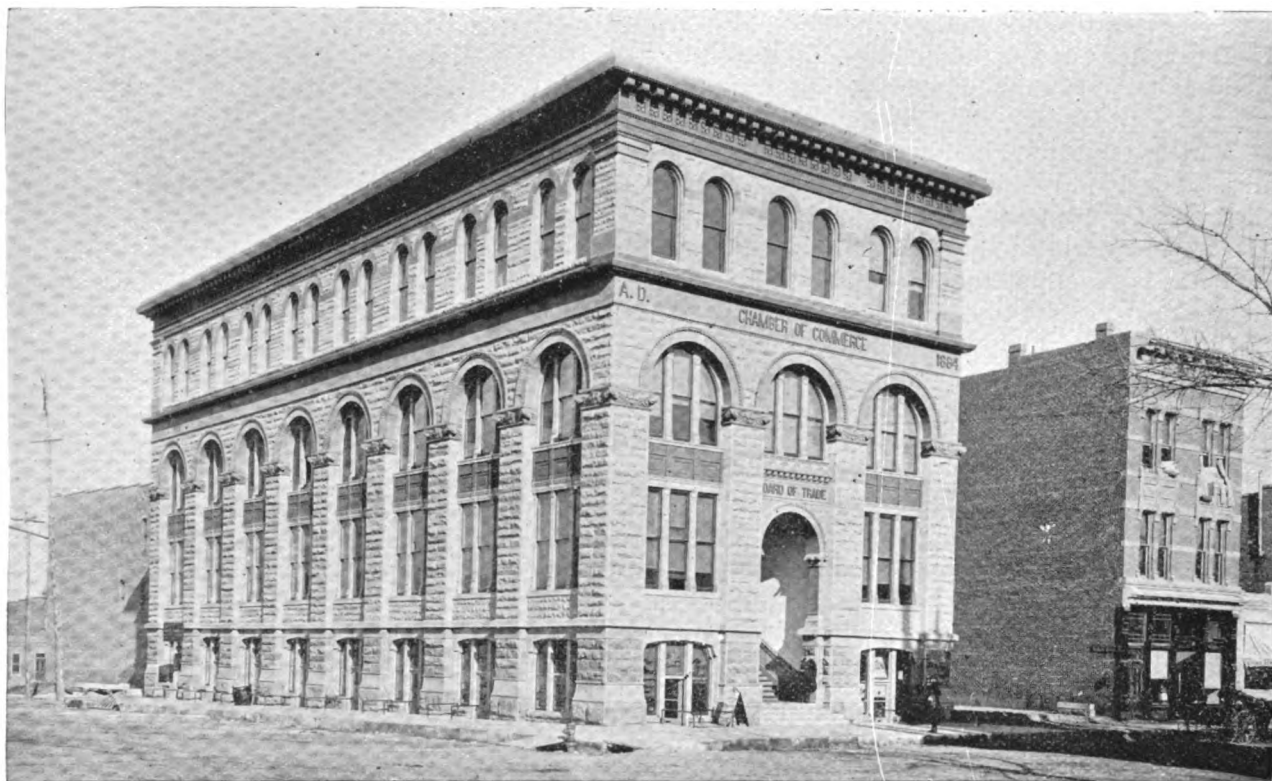
CHAMBER OF COMMERCE, DENVER. HOME OF THE BOURSE
