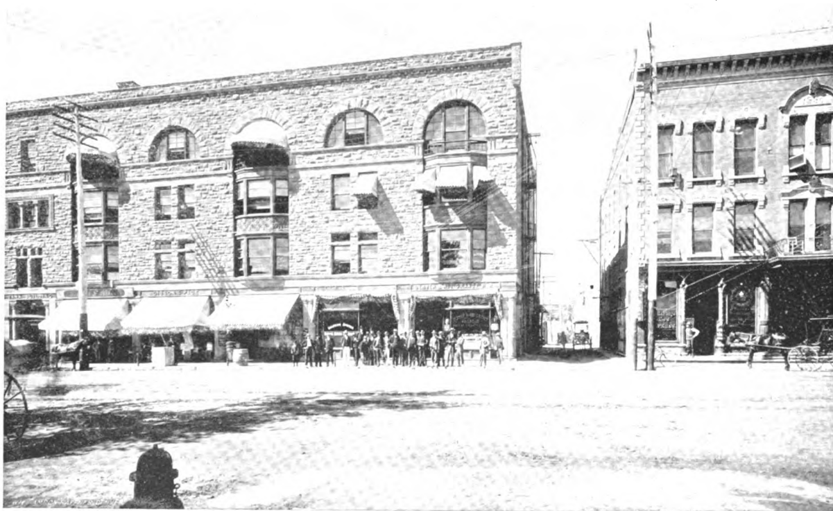
FIRST NATIONAL BANK BUILDING AND COLORADO SPRINGS STOCK EXCHANGE
