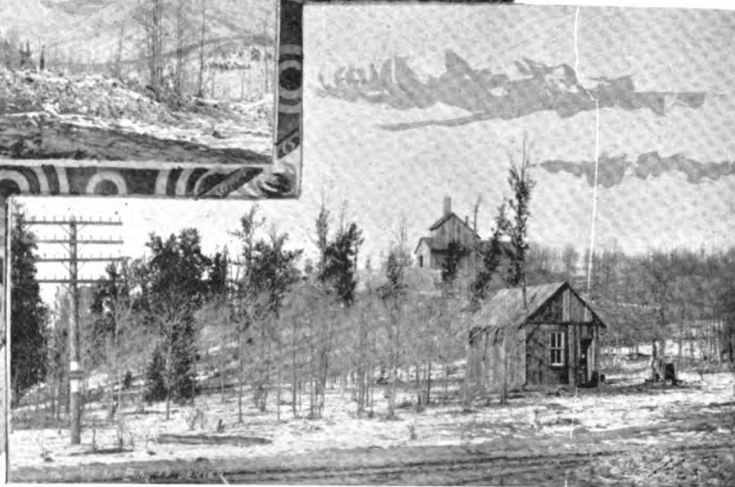
LONDONDERRY IRON CLAD HILL. NORTHEAST SLOPE.
