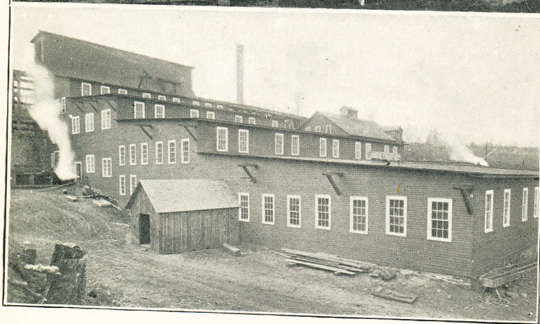
1. NO. 5 HOIST AT TAMARACK MINE. 2. TAMARACK STAMP MILL.
