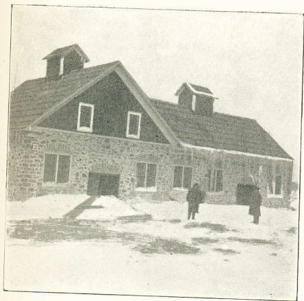
HOIST AND COMPRESSOR HOUSE, WOLVERINE MINE.
